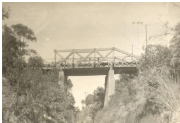
Plate 4: The former timber bridge on Dudley Rd in 1950. The missing members were damaged by termites. (Source LMCC #6646)
