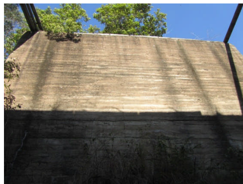
Plate 5: The eastern concrete headwall of the now demolished original timber bridge over the Fernleigh Track.
